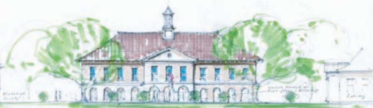
The proposed City Hall is raised on an elegant arcade-covered market. The non-habitable first floor below is designed to withstand flooding and can be used for a weekly farmers' market or to provide startup space for incubator businesses.
